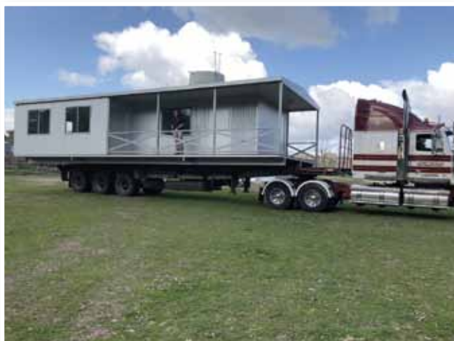
The new office for Ellerslie Park office arrives on a truck!
